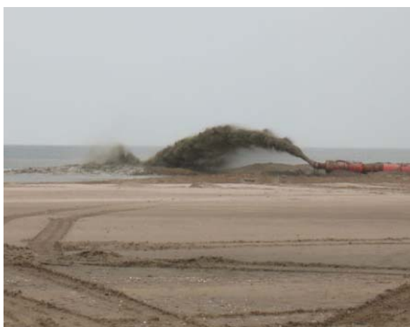
Dredging activities before the construction of Intake channel
